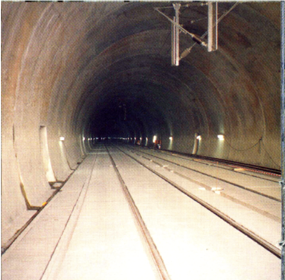
Figure 2. Embedded track systems for metro lines
